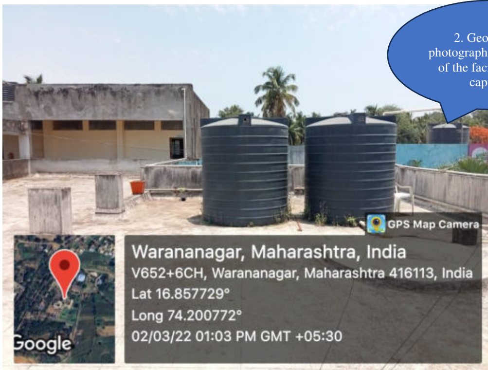
Water tanks of 5000 lit. capacity each.
